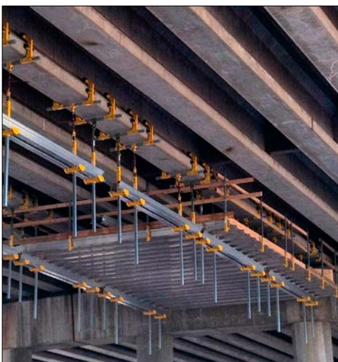
hanger, aluminum stringer & plywood deck set-up
