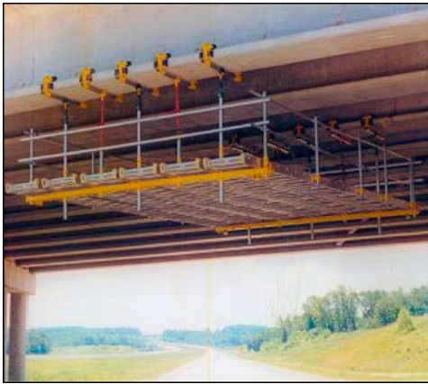
truss & aluminum stage set-up
