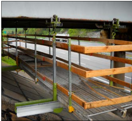
hanger, aluminum stringer & aluminum stage set-up
