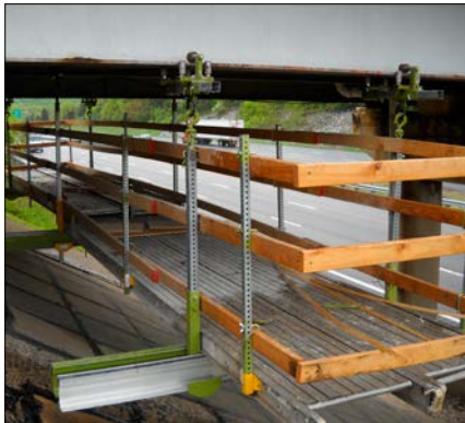
hanger, aluminum stringer & aluminum stage set-up
