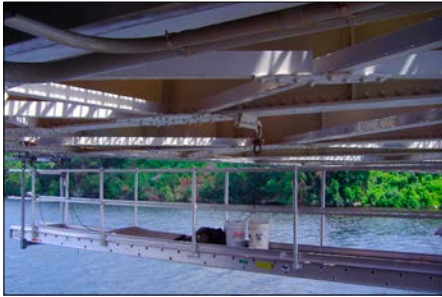
truss & aluminum stage set-up
