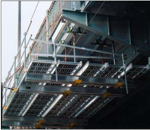
hanger, aluminum stringer & aluminum stage set-up
