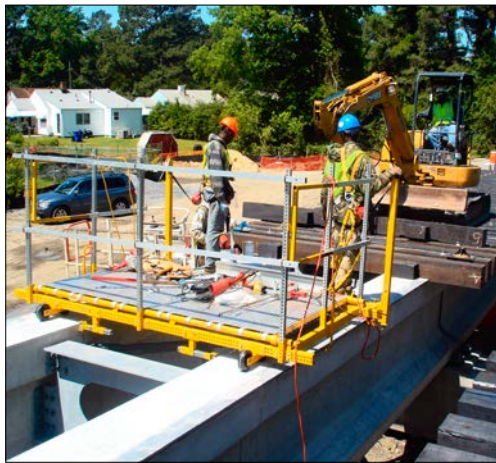
concrete girder application
