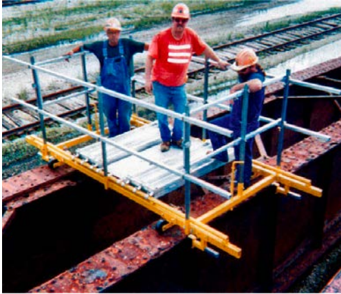
steel girder application
