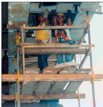
hanger, needle beam & scaffold plank set-up
