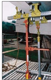
hanger, aluminum stringer & plywood set-up
