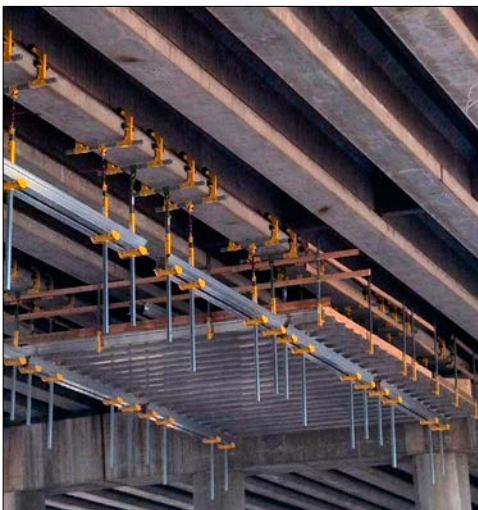
hanger, aluminum stringer & plywood deck set-up
